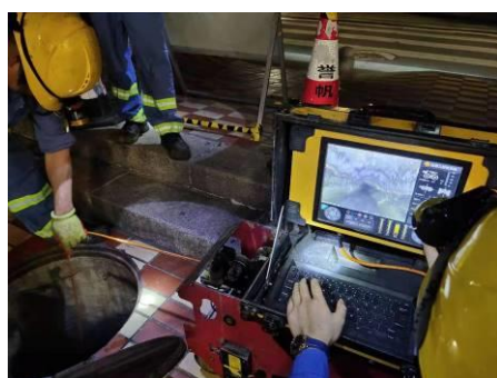
宜宾翠屏区检测现场
